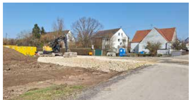
Baustelle Rennertshofen (Pumpstation)
